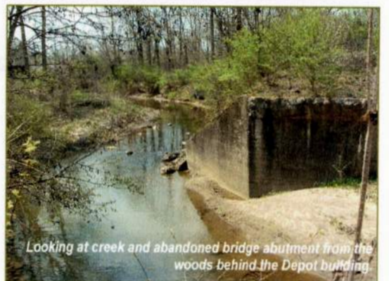
Looking at bridge over Six Mile Creek from Moser Park.
