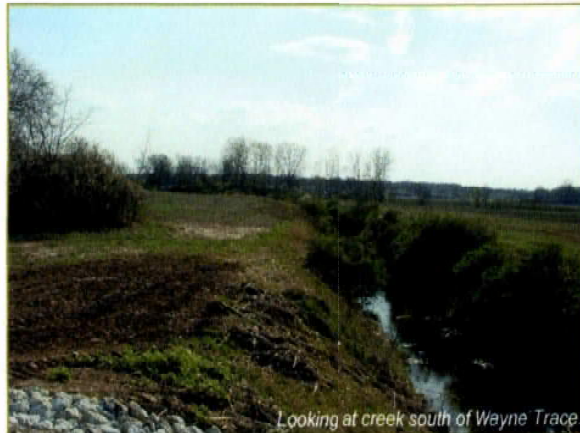
Looking south at new bridge carrying Wayne Trace over creek.
