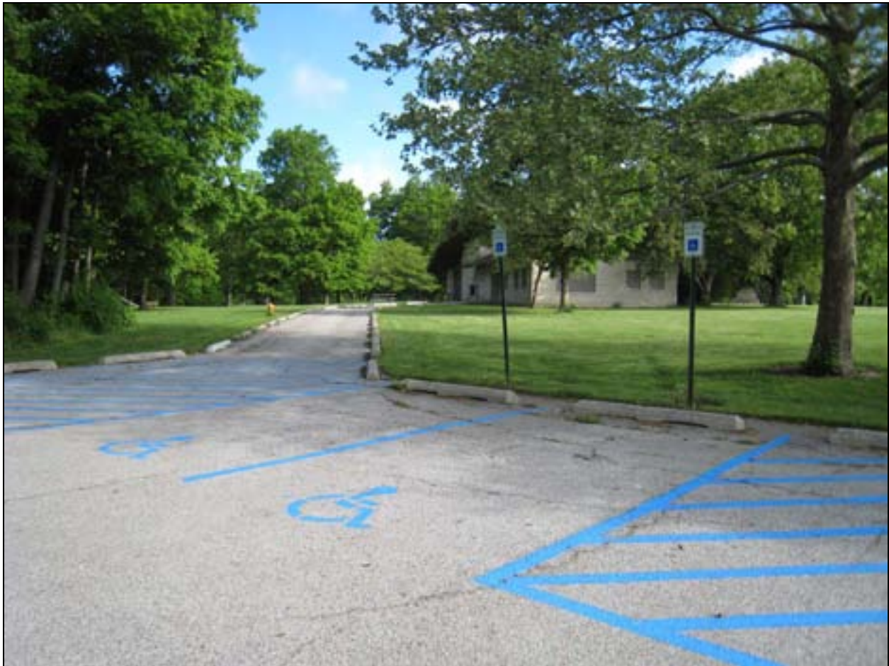
Figure IV.15 Concrete wheel stops mark the parking spaces in the lot south of the Conklin Pavilion and prevent vehicles from traveling onto the adjacent turf. A wide sidewalk connects the northwest corner of the parking lot with the pavilion entrance. Although the walk is wide enough to accommodate vehicles, it is restricted to pedestrian and service vehicle use only. Concrete wheel stops line the entire length of the sidewalk. (R-FWP-_20070517_0178.jpg) Courtesy Heritage Landscapes.
