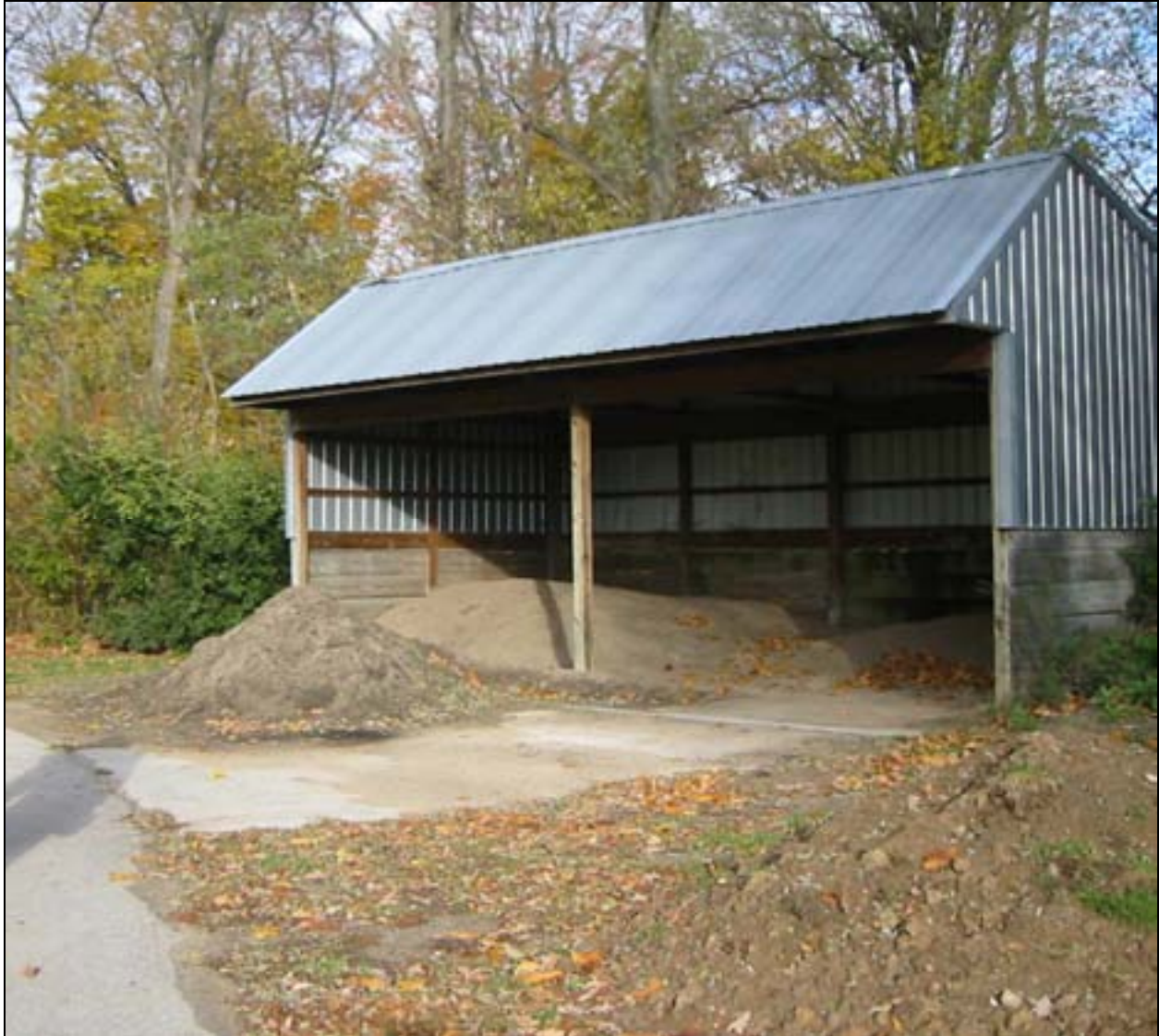
Figure IV.10 This maintenance shed is one of the structures located in Landscape Area 1. It is located along the northern half of the park loop drive, which is only accessible to pedestrians and maintenance vehicles. Constructed at the north edge of the area, the wood-frame shed has a metal roof and siding. The shed is used to store excess dirt. The open front makes it easily accessible by maintenance vehicles. (R-FWP-SHO-CT-(39).jpg) Courtesy Heritage Landscapes.
